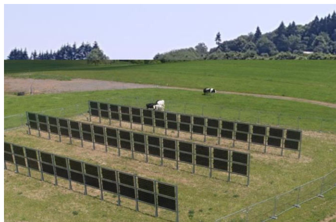
Figure 2.15. A 28 kW vertically installed bifacial PV system in Saarland, Germany.
