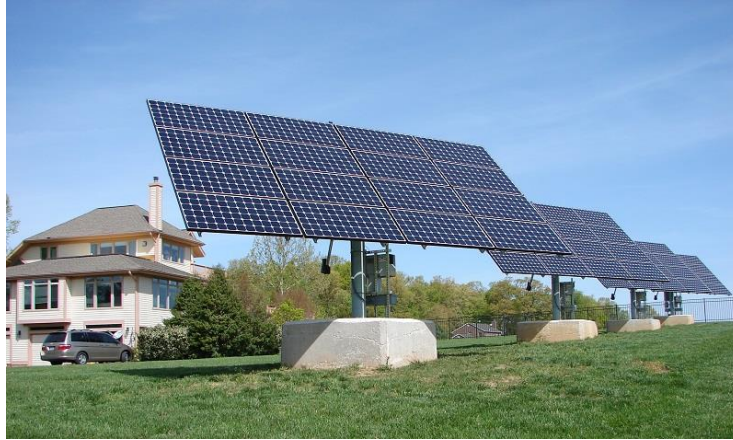
Figure 2.14. An example of two-axis tracking PV system. (Figure from www.aurorasolarenergy.com )
