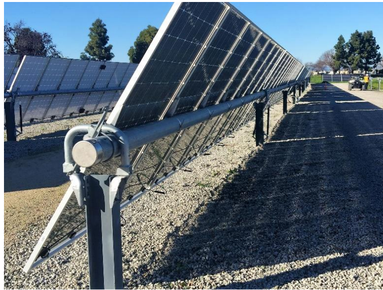
Figure 2.12. An example of a bifacial single-axis tracking PV system. (Image from www.NEXTracker.com )
